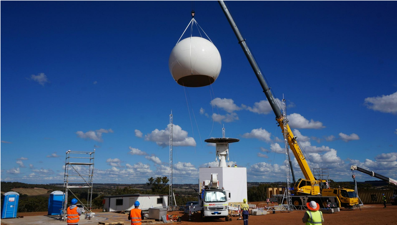
Transponder building with 5 m antenna on top of positioner and radome being installed
